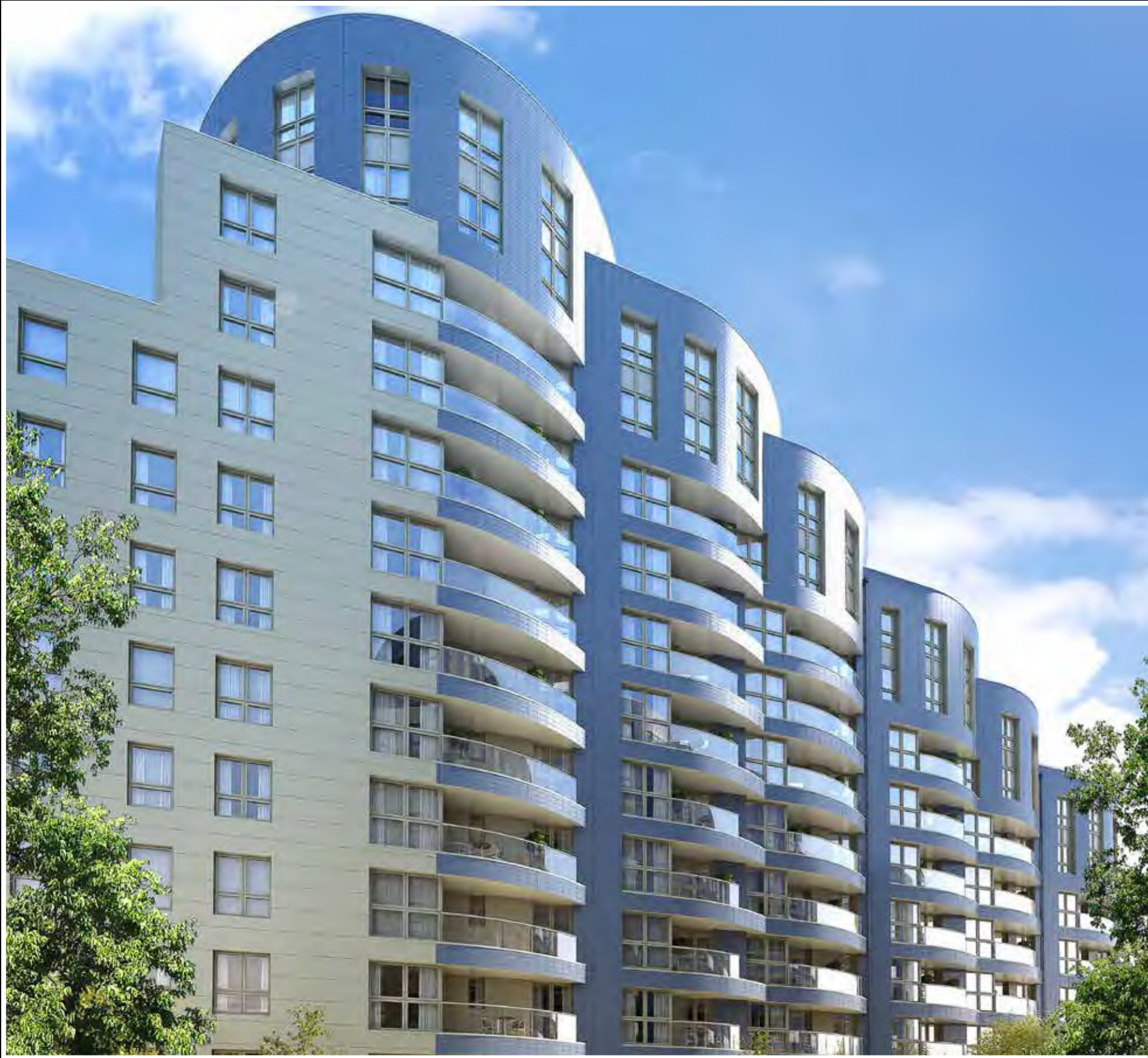
Gillespie Court, the final phase at Queensland Terrace.
